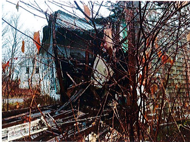
View of back of house where roof has totally collapsed, and the wall has also collapsed.
